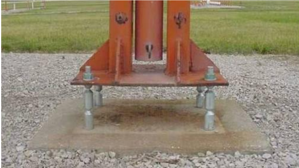
Figure 1. Application of fuse bolts
